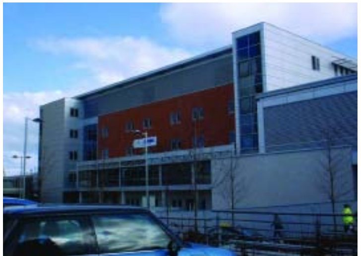
New Cancer Centre - Belfast City Hospital
