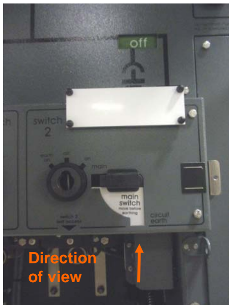
4.12 RSW2 Service position Main selected OFF
