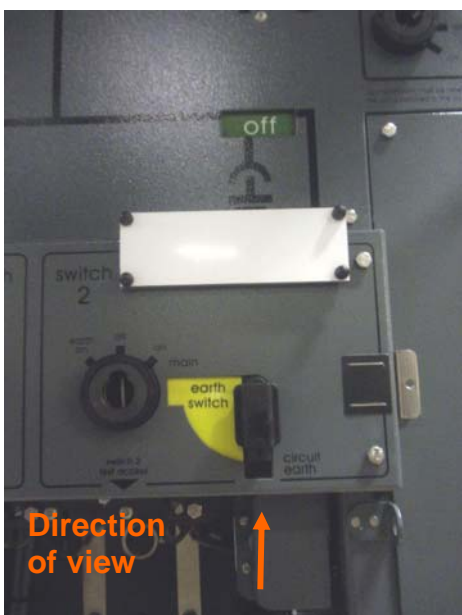
4.16 RSW2 Service position Earth selected OFF
