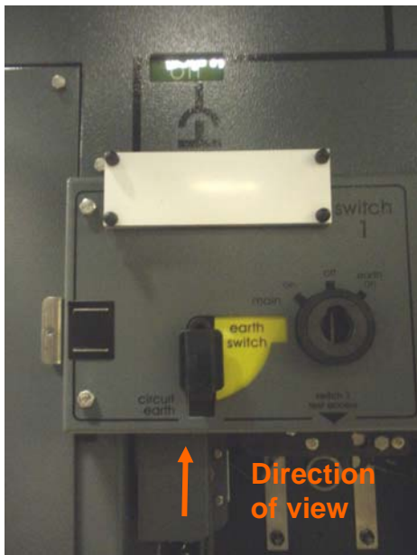
4.16 RSW2 Service position Earth selected OFF
