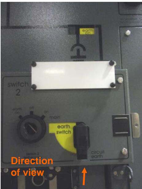
4.20 RSW1 Service position Earth selected Earth ON
