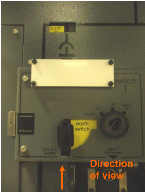
4.20 RSW1 Service position Earth selected Earth ON
