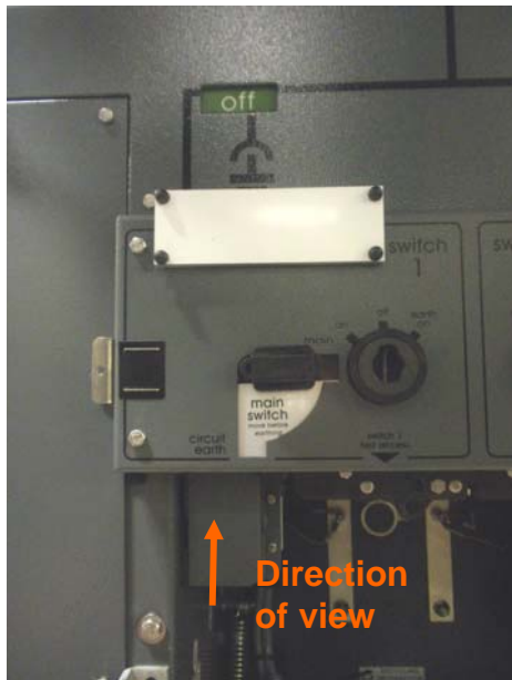
4.12 RSW2 Service position Main selected OFF
