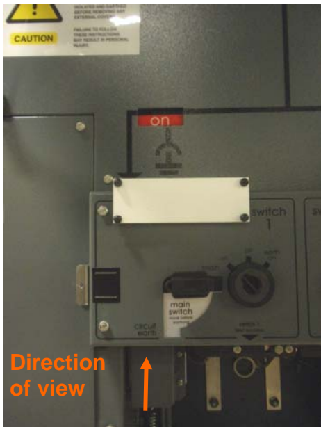
4.8 RSW2 Service position Main selected Main ON
